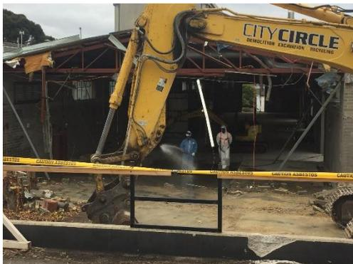
**Demolition of Building 32 with water spray to control dust**
