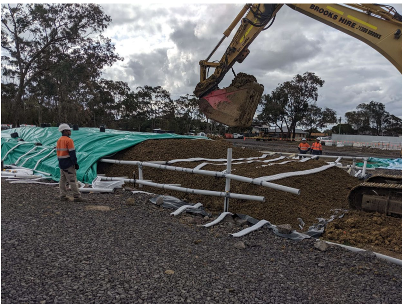
Formation of stockpiles with ventilation
