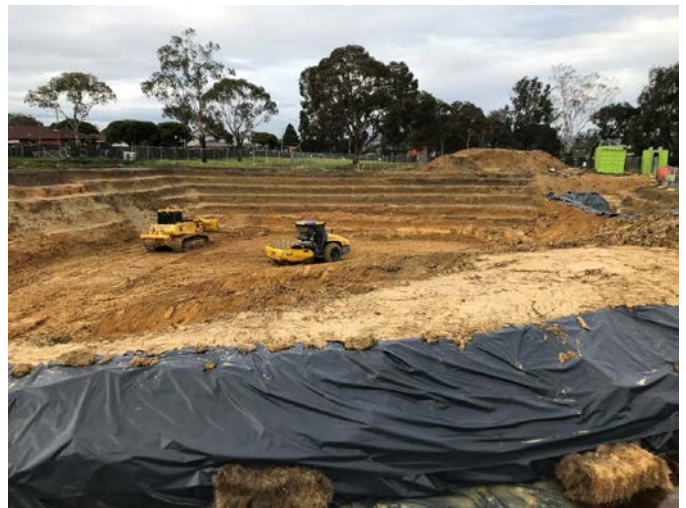
Backfilling and compaction in progress
