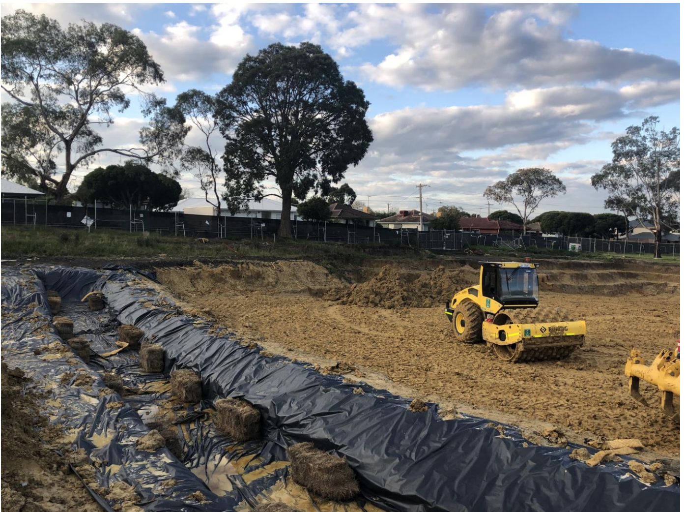
Compacting of soils in the pit during backfilling
