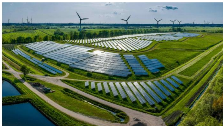
The new Electric Power Innovation for a Carbon-Free Society (EPICS) Centre will address challenges in clean energy production and storage.
