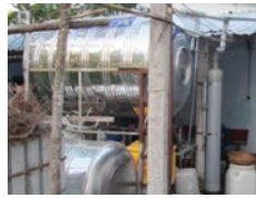
Rainwater harvesting system demonstration in a peri-urban household
